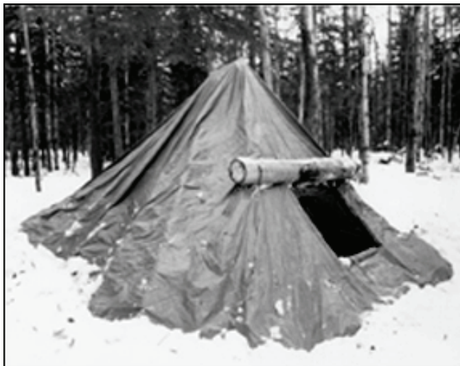
Figure 2-2. Covered frame of infrared counterdetection (thermal) shelter
