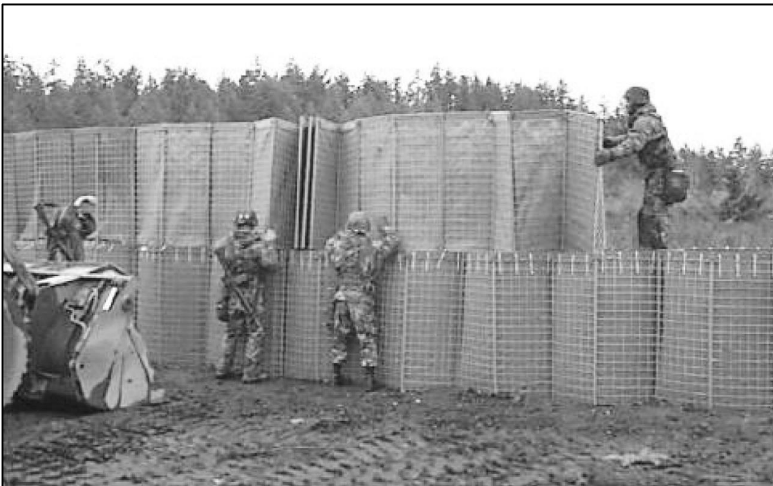
Figure 5-11. Wire and fabric container revetment
