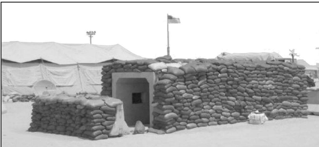
Figure 5-13. Properly sandbagged concrete shelter
